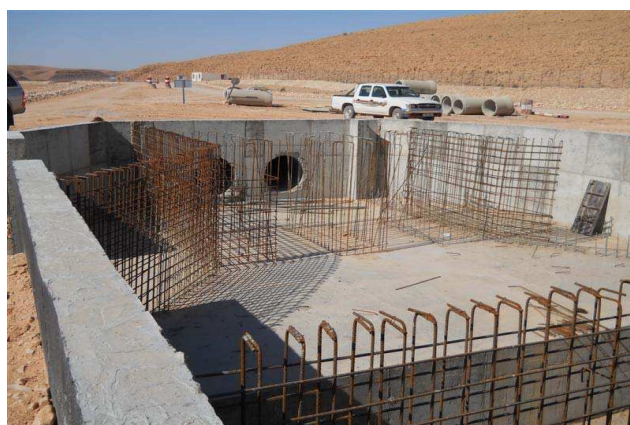
Figure 10 :Construction du RPTP
