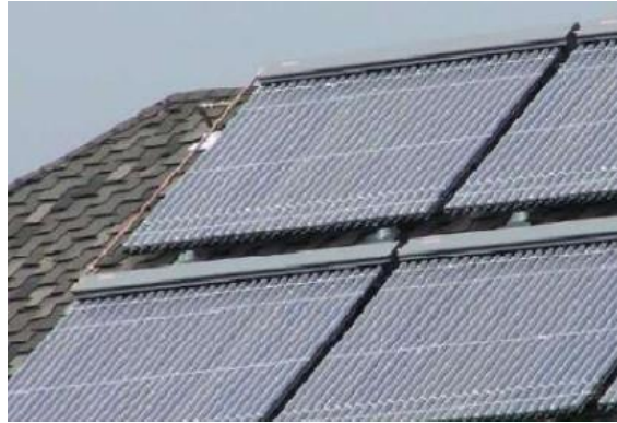
Figure II-8: Evacuated tube collector [2]
