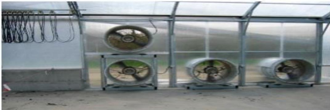
Figure 1-8 Ventilation forcée [14]
