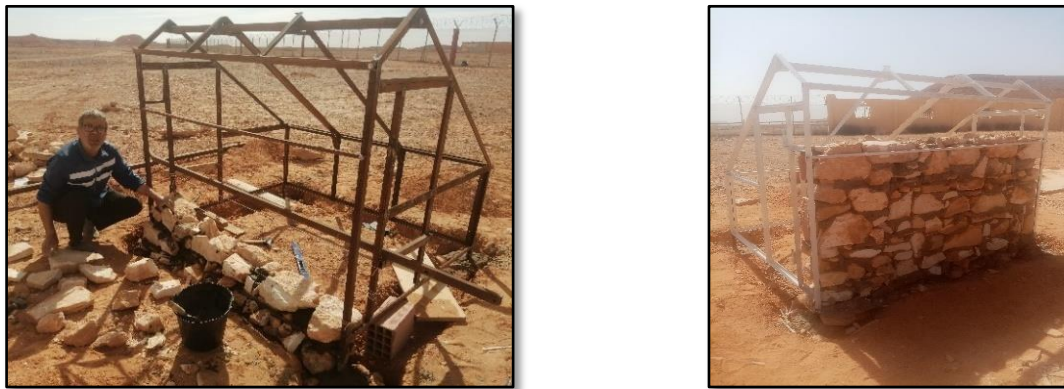
Figure III.10. On-site construction of the wall for the experimental greenhouse
