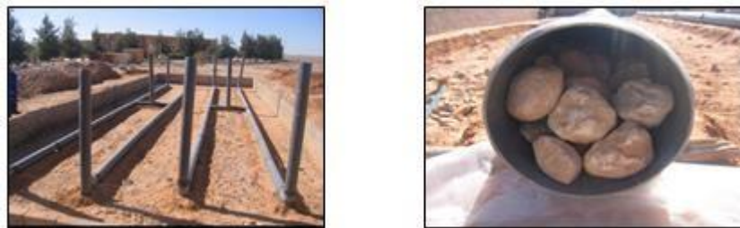
Figure II.4. Storage system based on a rock bed [9]
