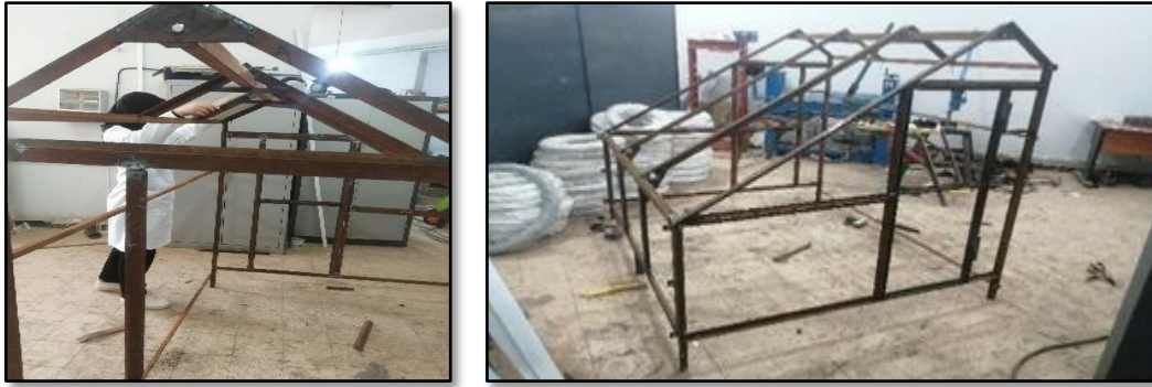
Figure III. 7. Greenhouse structure realization in atelier URAER
