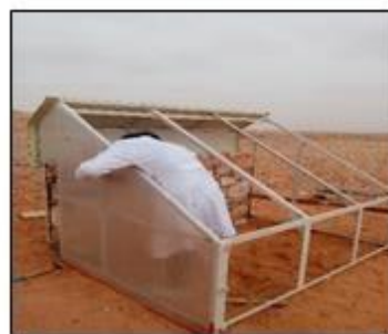
Figure III.12. Polycarbonate sheet installation
