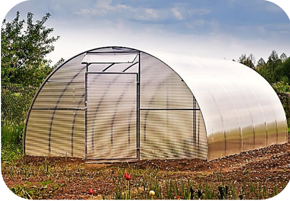
Figure I-12: Quonset Greenhouse [12].
