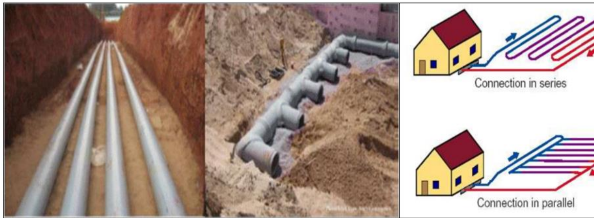
Figure I.7: Horizontal EAHE [13], [14]
