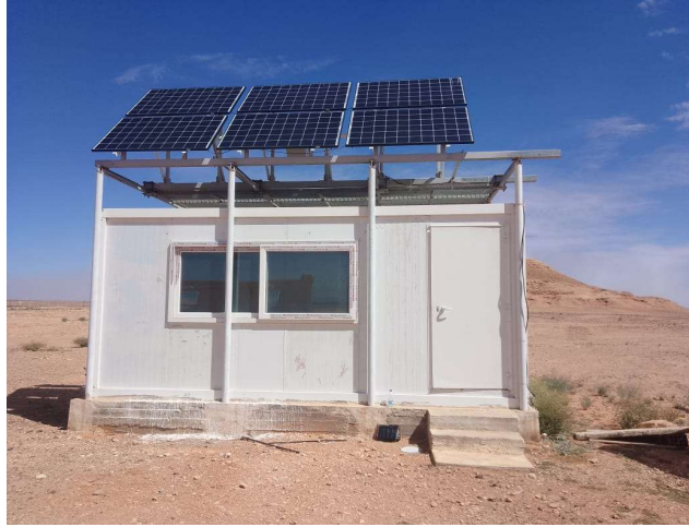
Figure 3-7: Outdoor view of the experimental building
