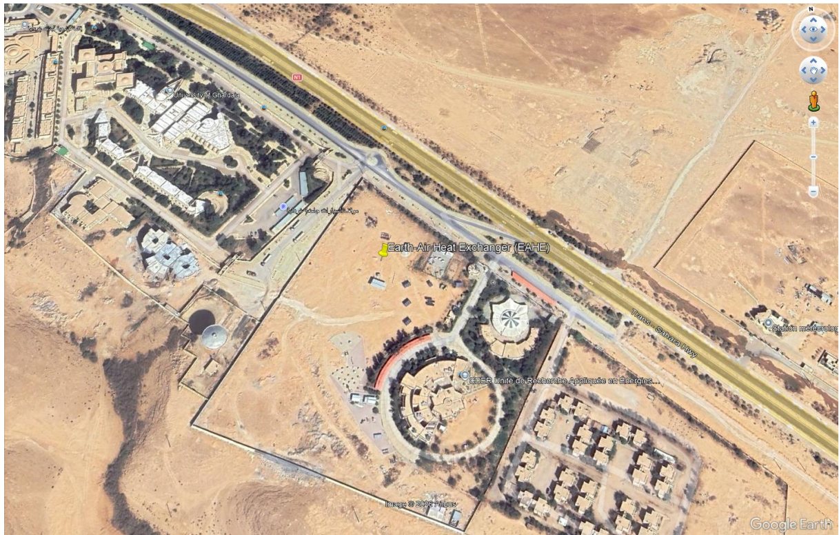
Figure 1-1: The Earth-Air Heat Exchanger (EAHE) installation site in Ghardaïa, Algeria [1].
