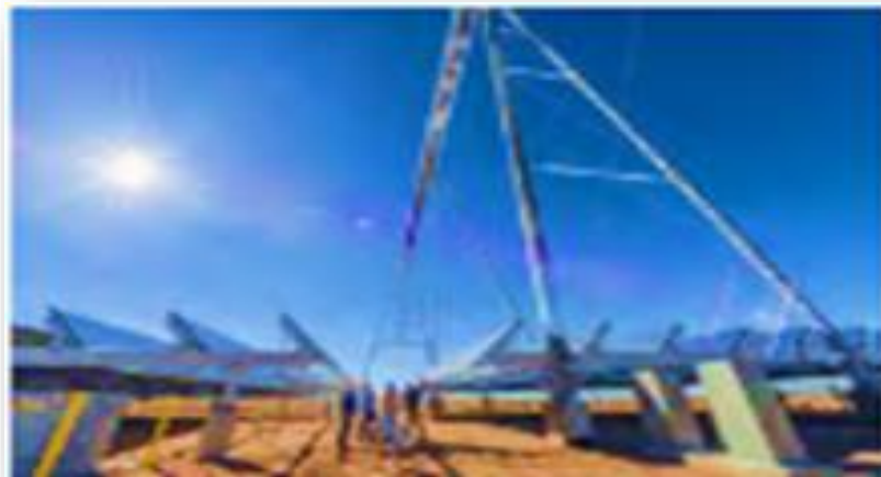
Figure (1-14): Fresnel concentrator.
