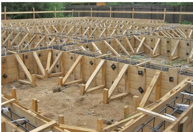
Fig 14: wooden formwork
