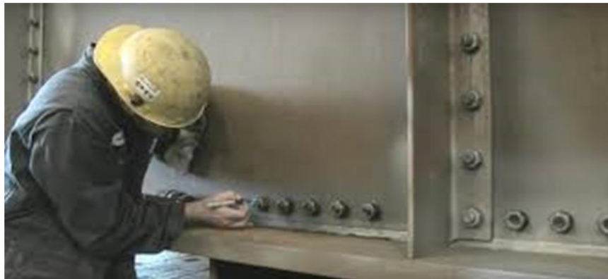
Figure 22 : Mechanical bolt assembly
