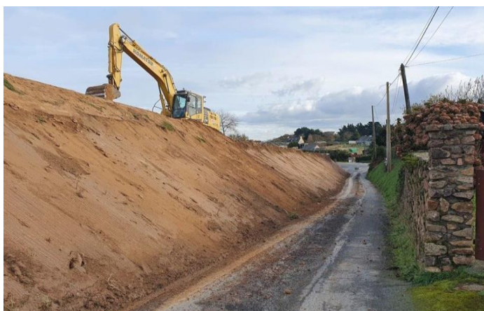
Fig 08: Embankment work
