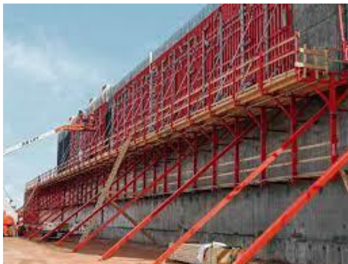
Fig 16: Climbing formwork
