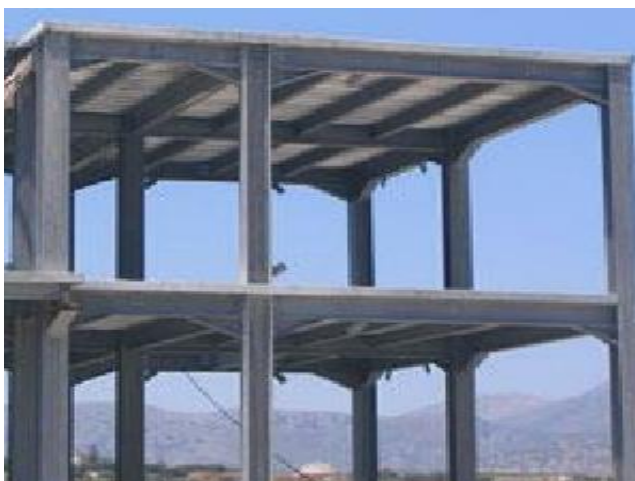
Fig 20 : The joining of sections with bolting
