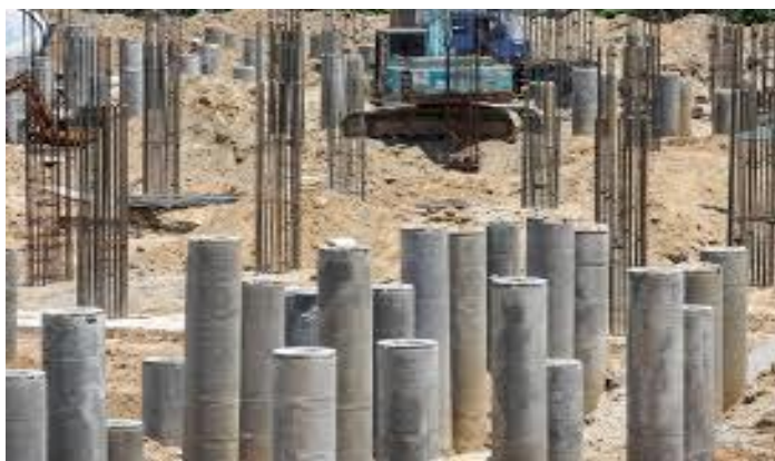
Fig 12: The deep foundations
