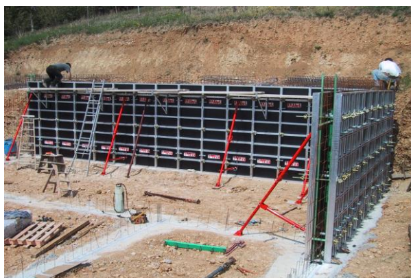
Fig 15: Metal formwork
