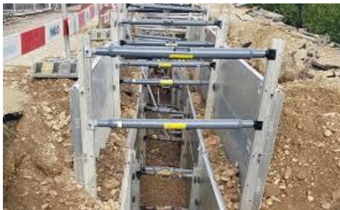
Fig 07: Slicing and shoring
