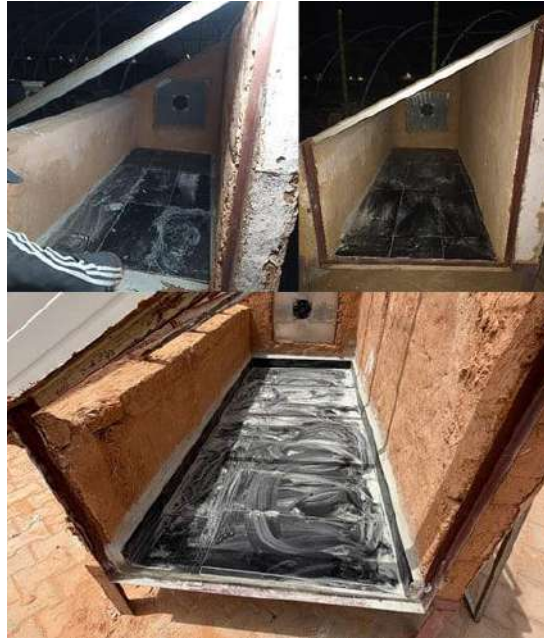
figure.II.11. the steps and results of installing floor tiles
