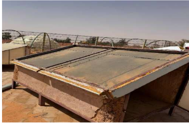
Figure III.4 Solar collector aluminum panel
