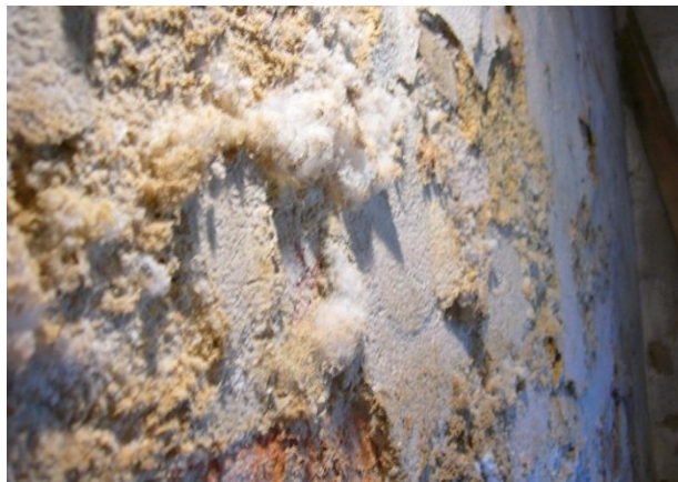
Figure 103 : Efflorescence [50]
