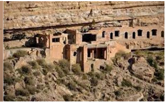
Figure 05 : Balcons "Govi" Aurasse [9]
