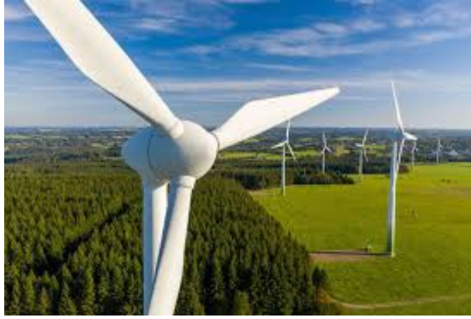
Figure 1.6: horizontal axis wind turbine.
