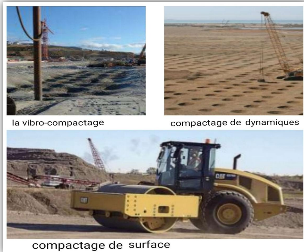
Figure N° 11: Les types de compactage[47]
