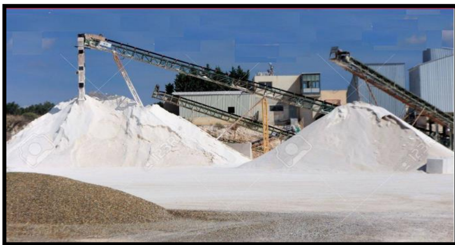
Figure (II.1): station de concassage.
