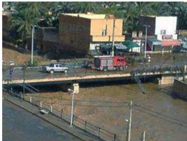
Figure III.2. L'oued Metlili en crue (Crue 12-13 /03/2011 Débit max = 570m 3 /s)(Photo. Ouled Belkhir, 2011)
