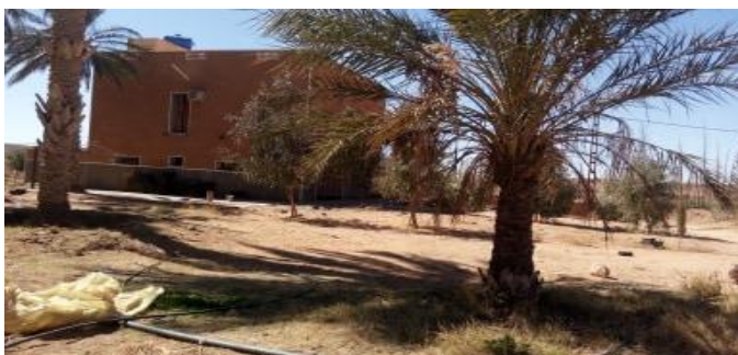
Station de Sidi Mebarik
