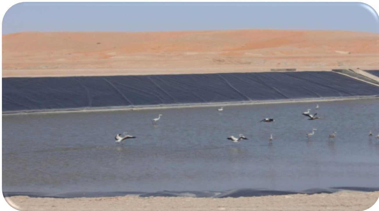
Figure 72.IV: Bassin de maturation
