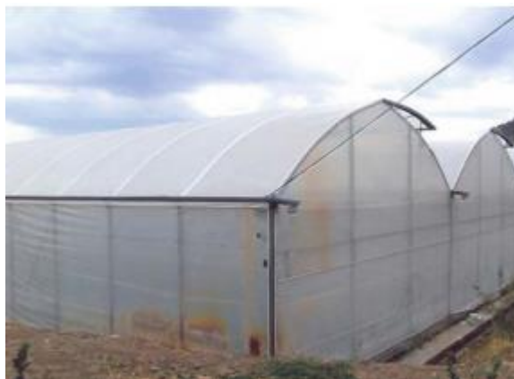
Fig. I. 10. Multi-span pointed-arched greenhouses.
