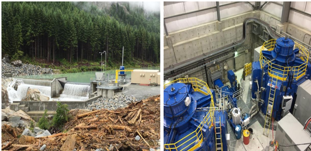
Figure 1.6: Jimmie Creek Hydroelectric Project [17]
