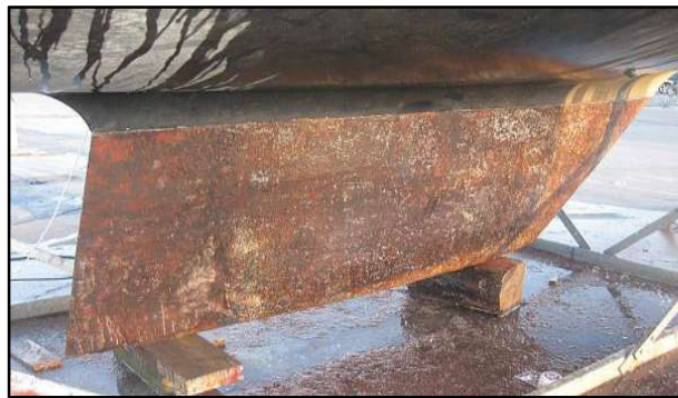
Figure 3 : corrosion galvanique [B]
